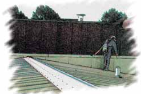
A complete system consists of the saferidge section, endstops, traveling eyebolt, a full body harness, and a rope grab.
