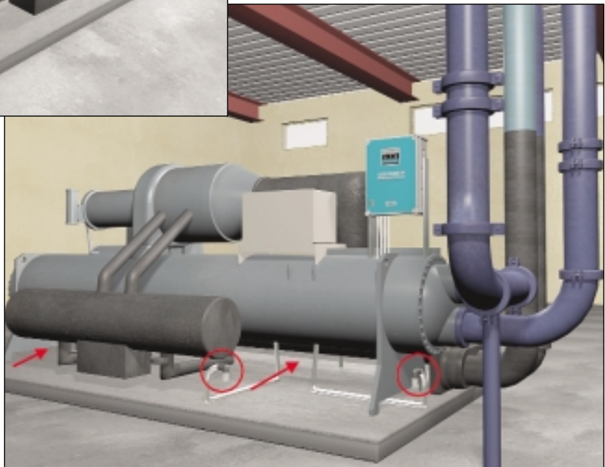
Figure 4: A Chillgard LE Monitor is located in the mechanical room providing integrated sensing and controlling. Up to four points of monitoring provide for maximum protection around the chiller.
