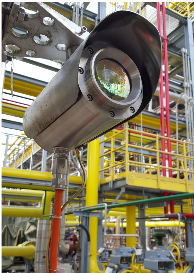
Figure 2. Senscient ELDS™ laser-based open path gas detector (OPGD).
