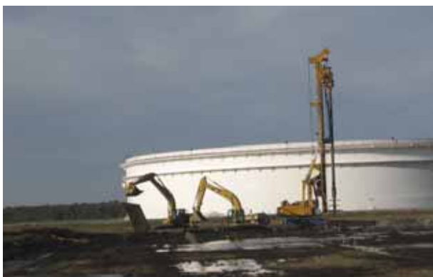
Figure 5. Soil mixing carried out at the project site.
