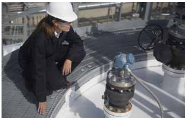
Figure 3. A Rosemount 5300 guided wave radar level transmitter on a sphere tank in a gas processing plant.
