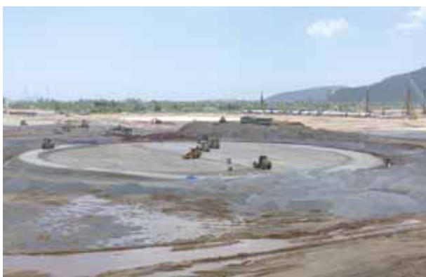
Figure 6. Completion of the perimeter ring berm.
