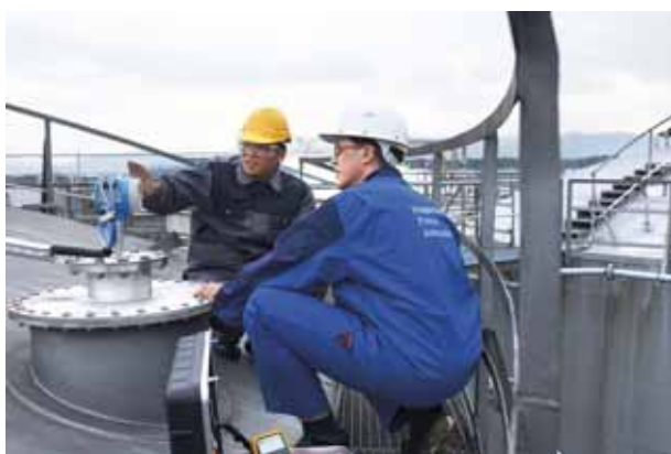
Figure 5. Radar level instruments have the necessary accuracy for custody transfer applications.
