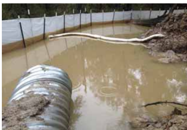
Figure 2. Deployment of spunbond nylon fabric used to contain spilled oil in Mooringsport, Louisiana.
