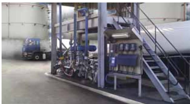
Figure 5. Terminal and storage facility in UK with meters and overfill/earthing control unit on the gantry.
