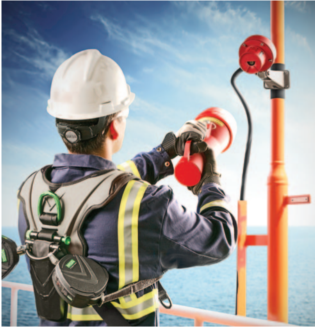
Fig. 3 – Flame detector being tested with test lam.
